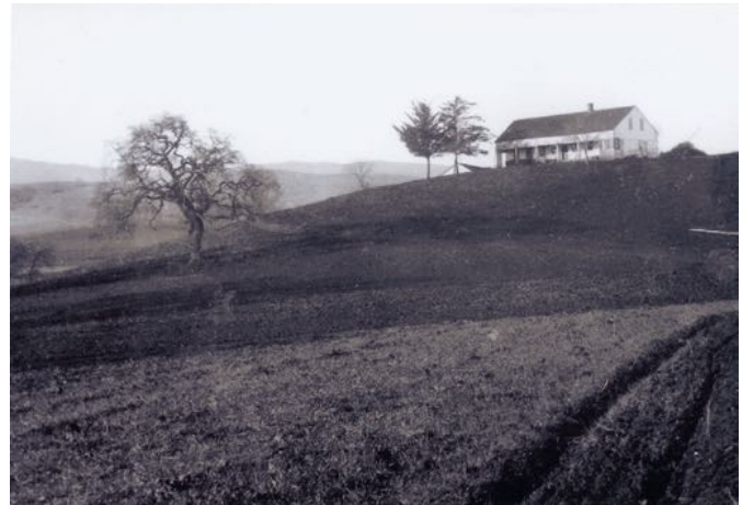
Juana Briones’ mid-1840s home, a rare construction of earthen adobe material encased inside wooden framing, sat at the end of today’s Old Adobe Road in the Los Altos hills. Courtesy California Historical Society.
