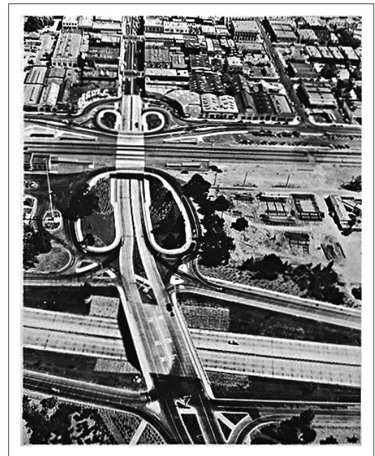
The University Avenue underpass, 1941, viewed from Stanford looking east towards downtown (Guy Miller Archives online).
